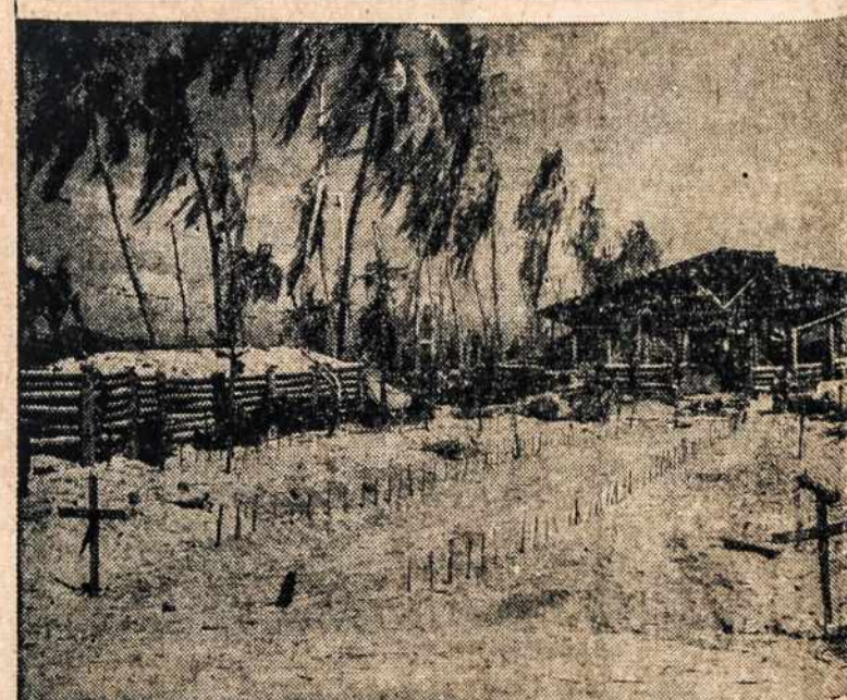
The wrecked building (right background) was a Japanese administration building on Tarawa before the bombs and shells started to fall and Marines land. The bomb-proof shelter (left) was for use of the officers who fled the building.
